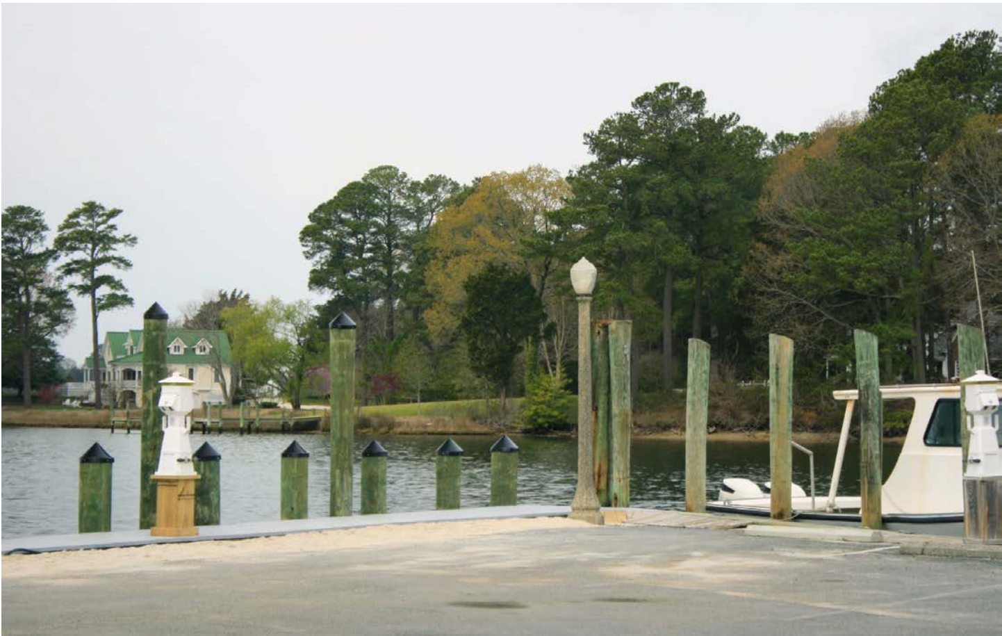
The existing wharf
