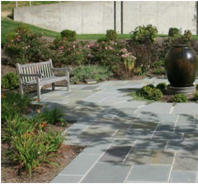
Example of Bluestone Paving Terrace
