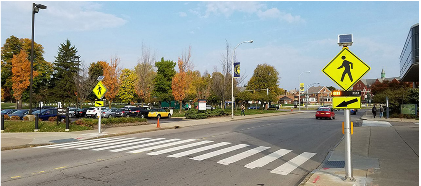
Pedestrian-activated rectangular rapid flashing beacon (RRFB) signs offer a higher level of awareness to the driver at crossing locations. These signs have strobes that are activated when pedestrians wish to cross the street by pushing a button. They can also be activated in a passive manner using thermal imaging so that they activate whenever a pedestrian approaches the crosswalk. The fact that these are dark until activated and not constantly flashing offers a higher level of warning to the drivers of pedestrian crossing activity.
